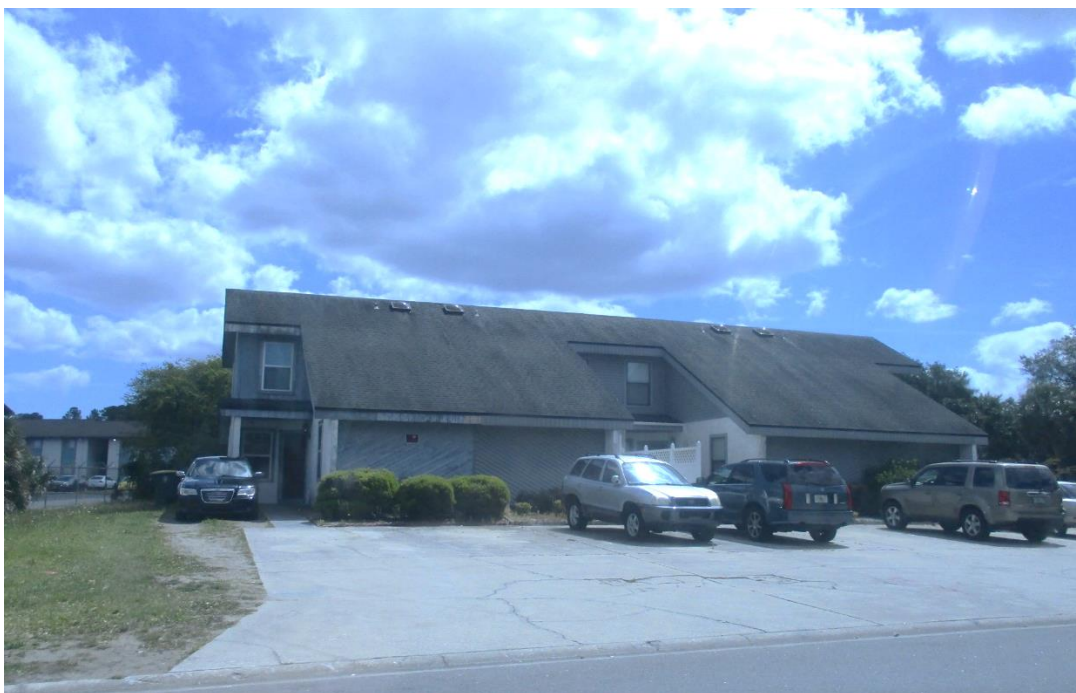
View of Property to the South
